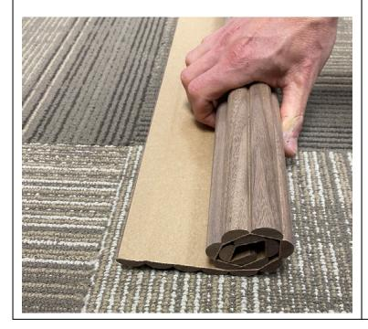
Bend tambour panel to the outside. Use a good amount of force to really flex the panel and stretch out the paper
